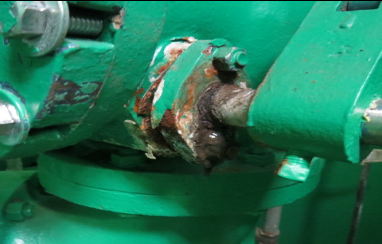
Photograph #: 19 Date: January 12, 2016 – Lift Station #4 (Buffalo, MN) Subject: Close up view of leaking valve
