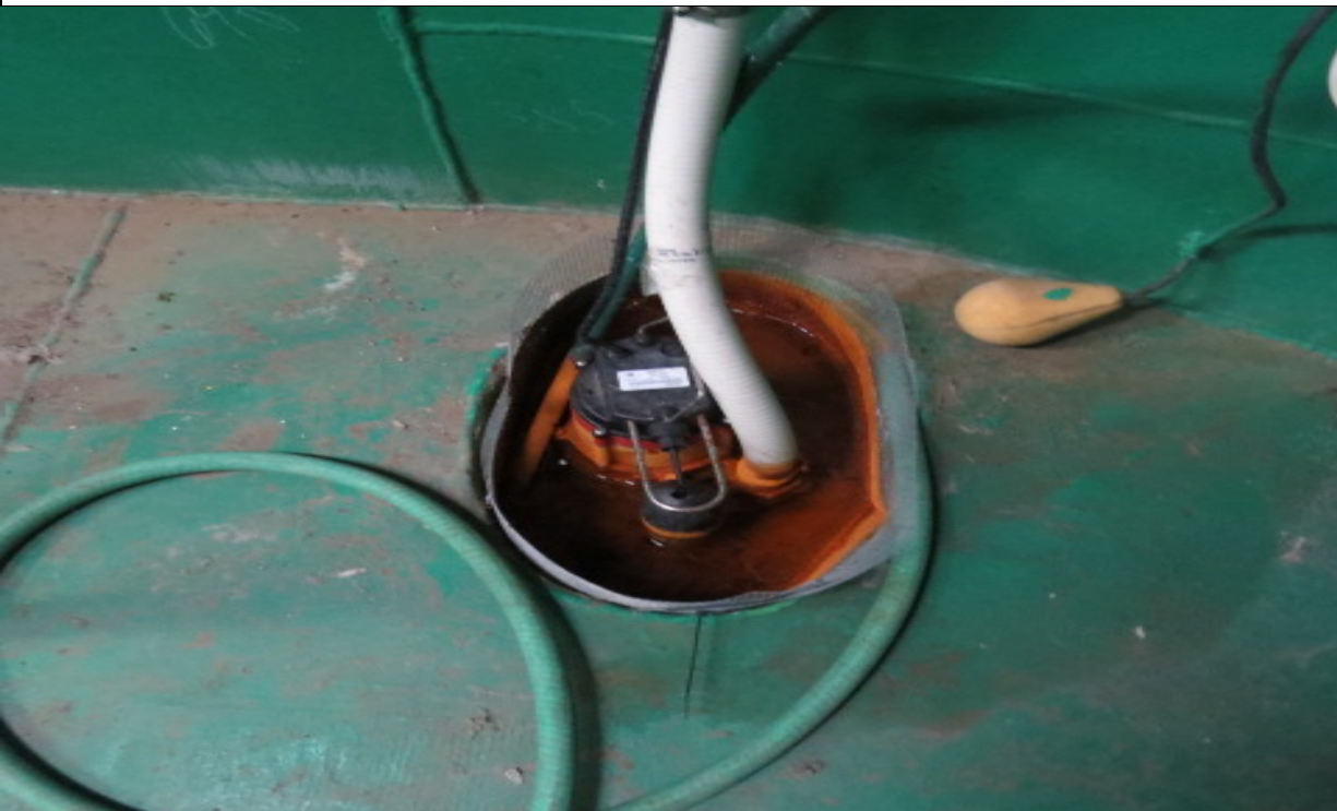
Photograph #: 16 Date: January 12, 2016 – Lift Station #4 (Buffalo, MN) Subject: View of sump pump
