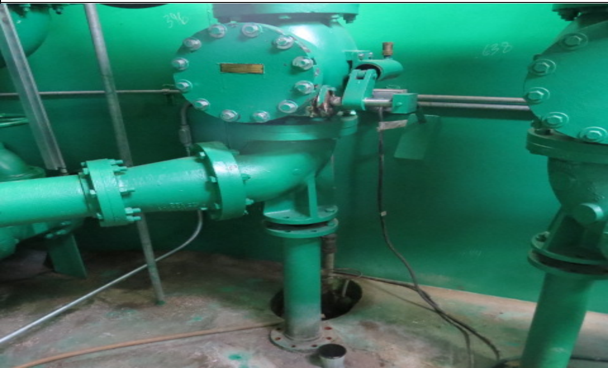
Photograph #: 18 Date: January 12, 2016 – Lift Station #4 (Buffalo, MN) Subject: View of sump pump and leaking valve
