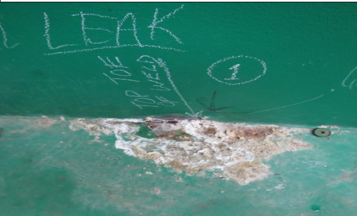
Photograph #: 10 Date: January 12, 2016 – Lift Station #4 (Buffalo, MN) Subject: Area of leak #1 (note: evidence of active leak)
