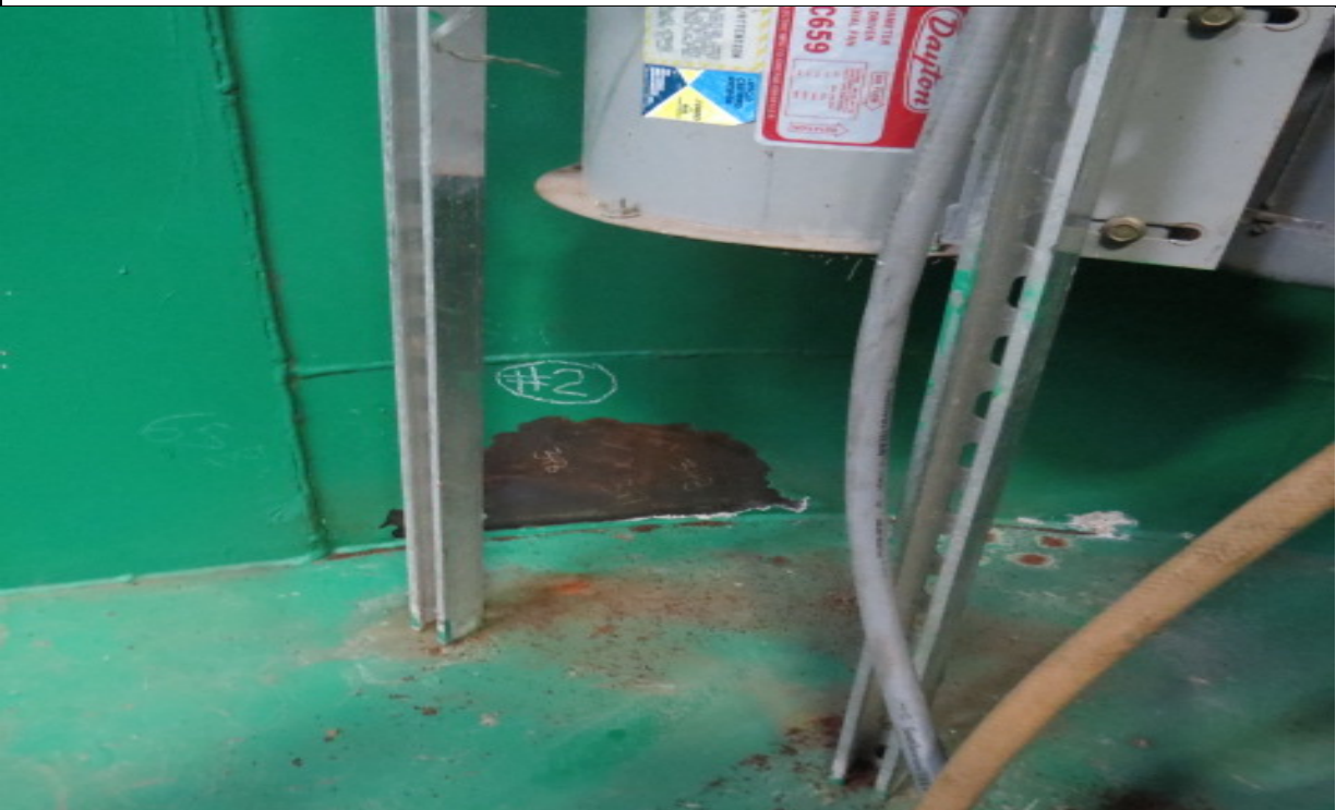
Photograph #: 12 Date: January 12, 2016 – Lift Station #4 (Buffalo, MN) Subject: View at area of “possible “ leak #2
