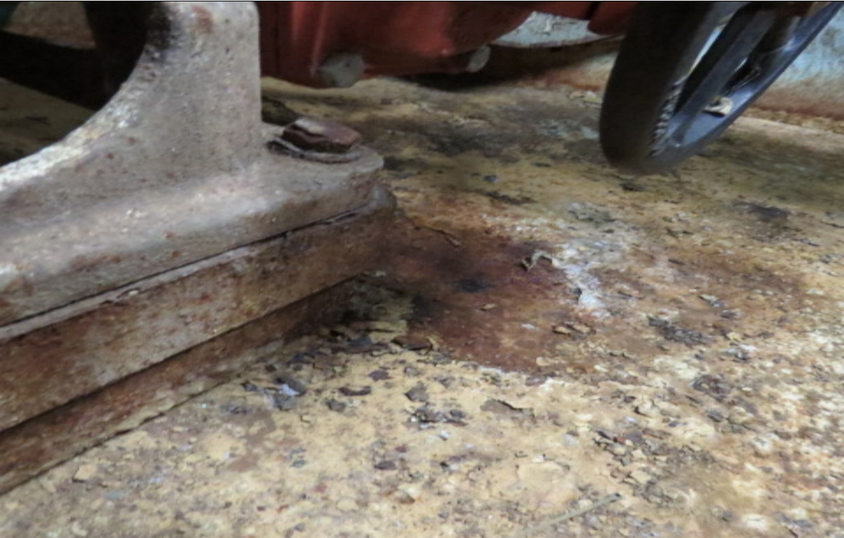
Photograph #: 7 Date: January 12, 2016 – Lift Station #3 (Buffalo, MN) Subject: Close up view of chamber floor corrosion
