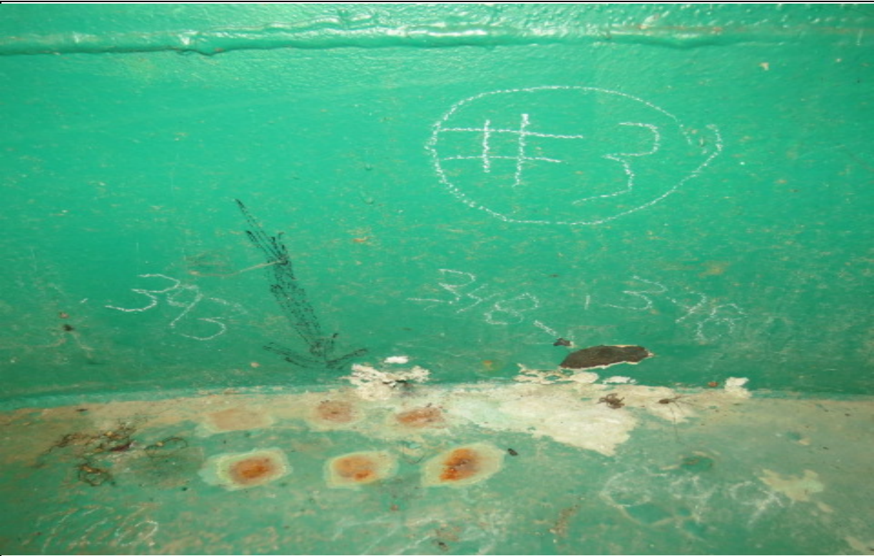
Photograph #: 15 Date: January 12, 2016 – Lift Station #4 (Buffalo, MN) Subject: View at area of “possible “ leak #3
