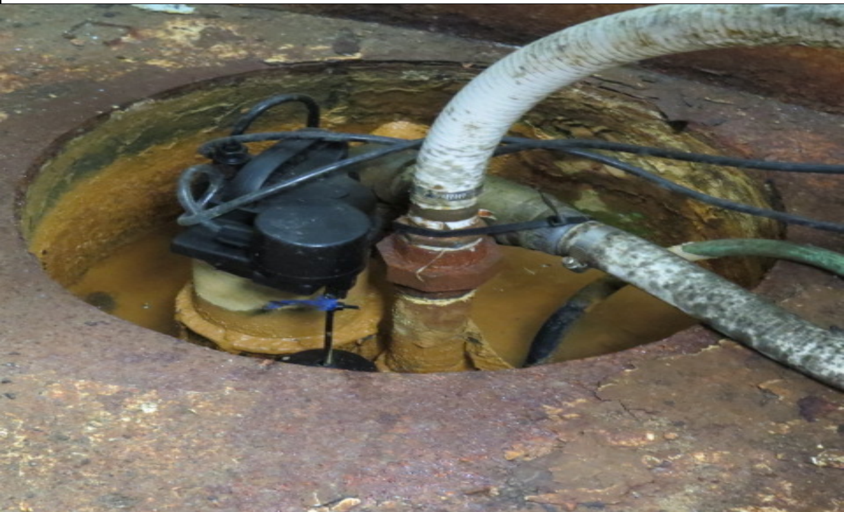
Photograph #: 6 Date: January 12, 2016 – Lift Station #3 (Buffalo, MN) Subject: View of sump pump
