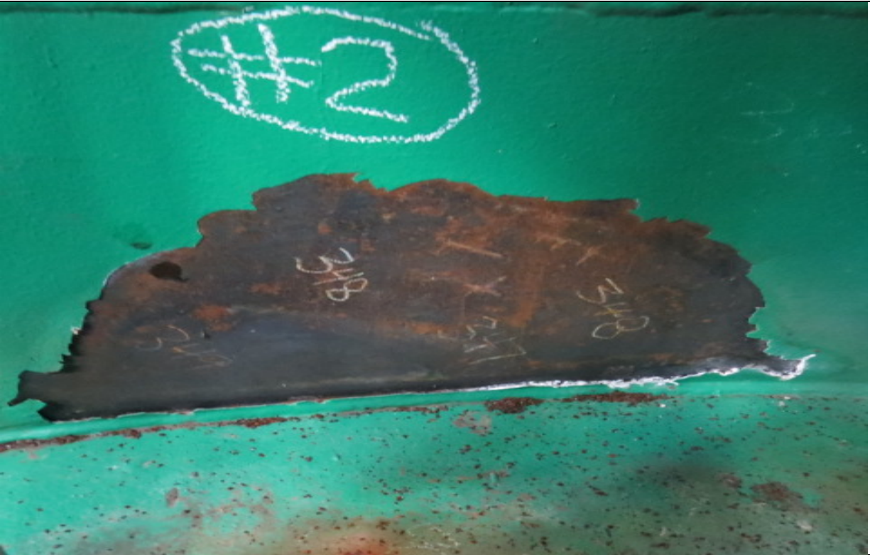
Photograph #: 13 Date: January 12, 2016 – Lift Station #4 (Buffalo, MN) Subject: Close up view of “possible “ leak #2
